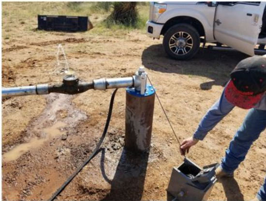
Pump Testing on Well CSA 1
